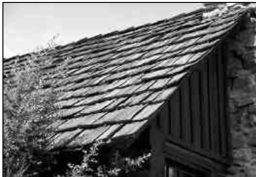
Flammable wood shingles frustrate fire fighting efforts and exacerbate property losses (Photo: Bureau of Land Management)
